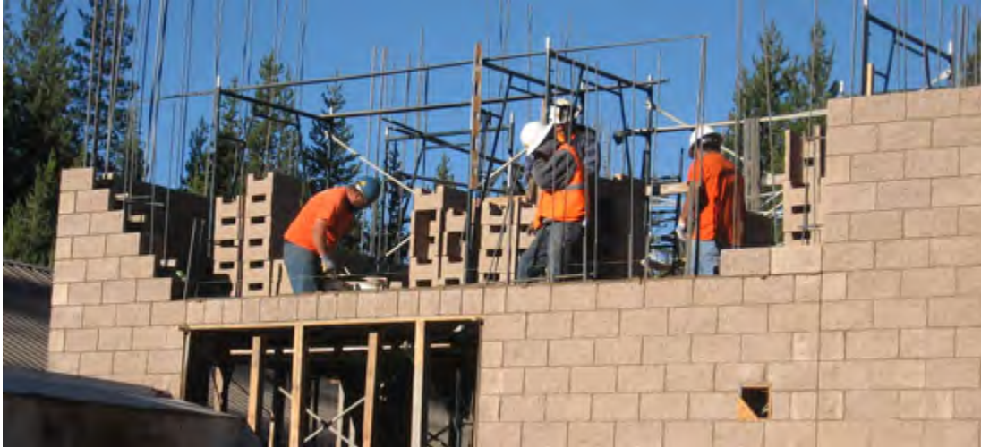
Constructing brick walls at the MBR building
